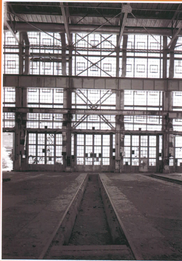
Erecting bay pit, doors, window wall
