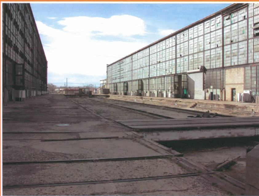
Machine Shop (L) & Boiler Shop (R) looking west. The Transfer Table allowed east-west transfer of engines on a site where all tracks run north-south, and bridged between the Machine and Boiler shops.
